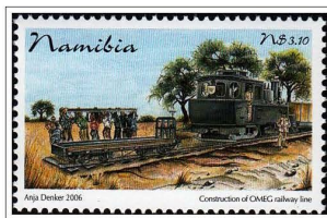
Construction of OMEG railway line
